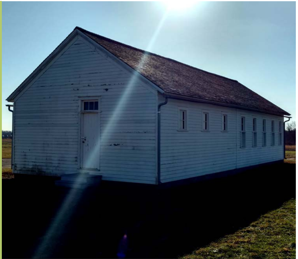
Asylum during the inspection on December, 27th 2016
