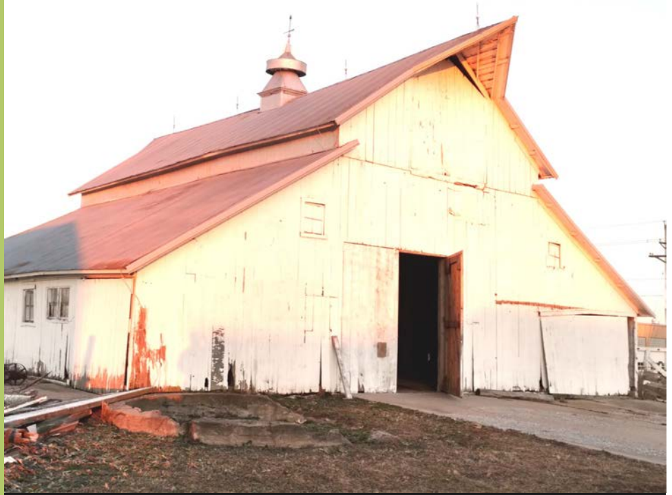
West Barn during the inspection on December 27th, 2016
