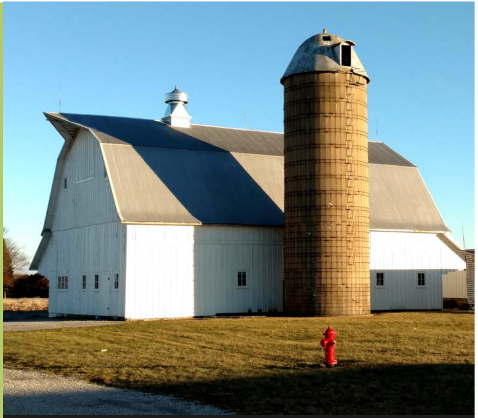
Dairy Barn during the inspection on December 27th, 2016.
