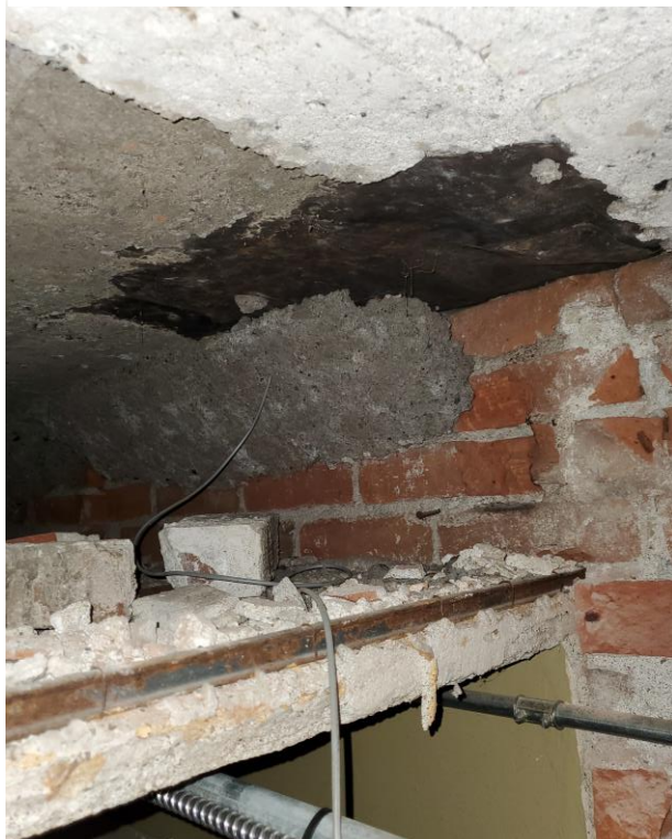
Plaster ceiling intersecting masonry wall.
