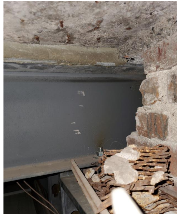
Steel beam penetration through masonry wall.
