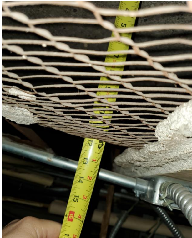
Wire mesh and plaster ceiling.
