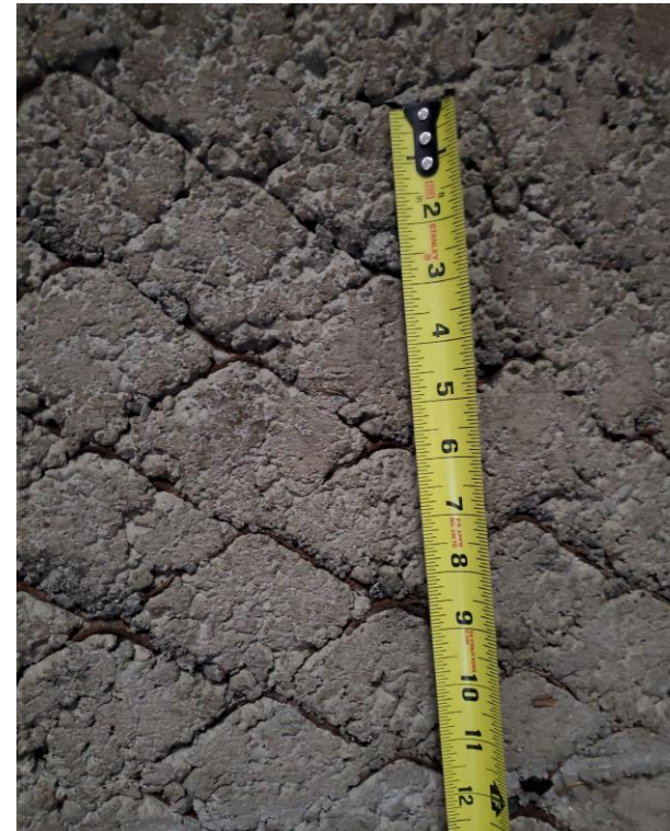
Wire mesh in concrete slab.
