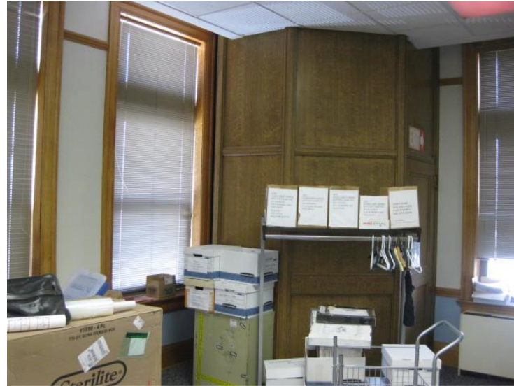
Clerk of Courts - SW stair enclosure.
