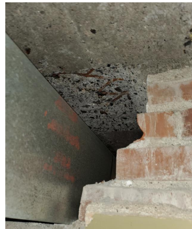
Ductwork penetration through masonry wall.
