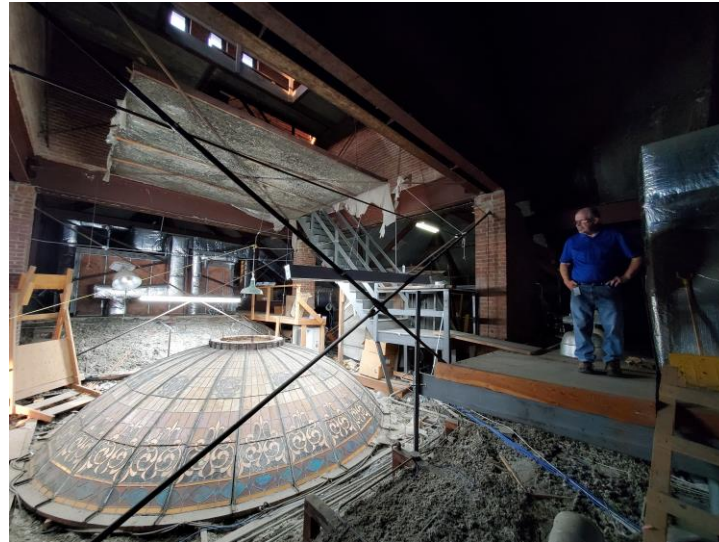
Glass dome above lobby in attic.
