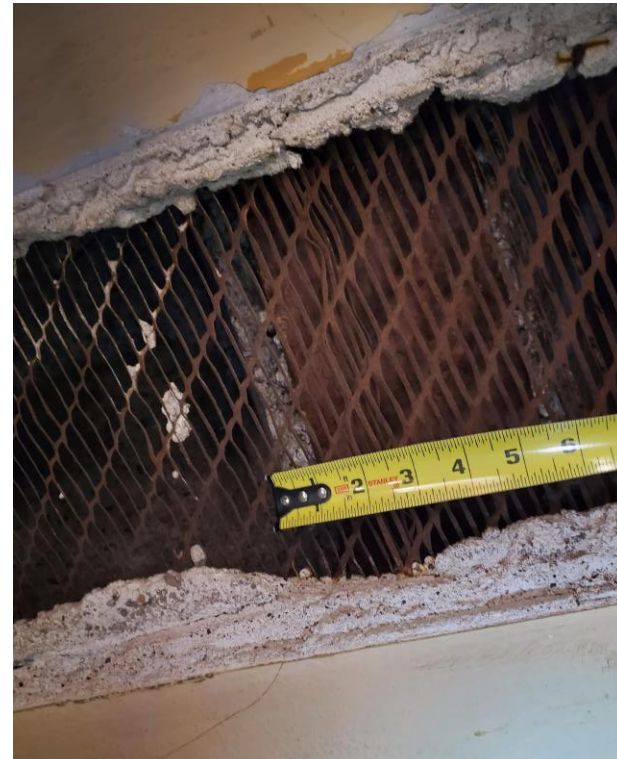
Wire mesh and plaster ceiling.
