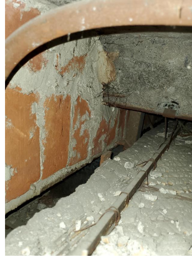
Beam intersecting wall and plaster ceiling.
