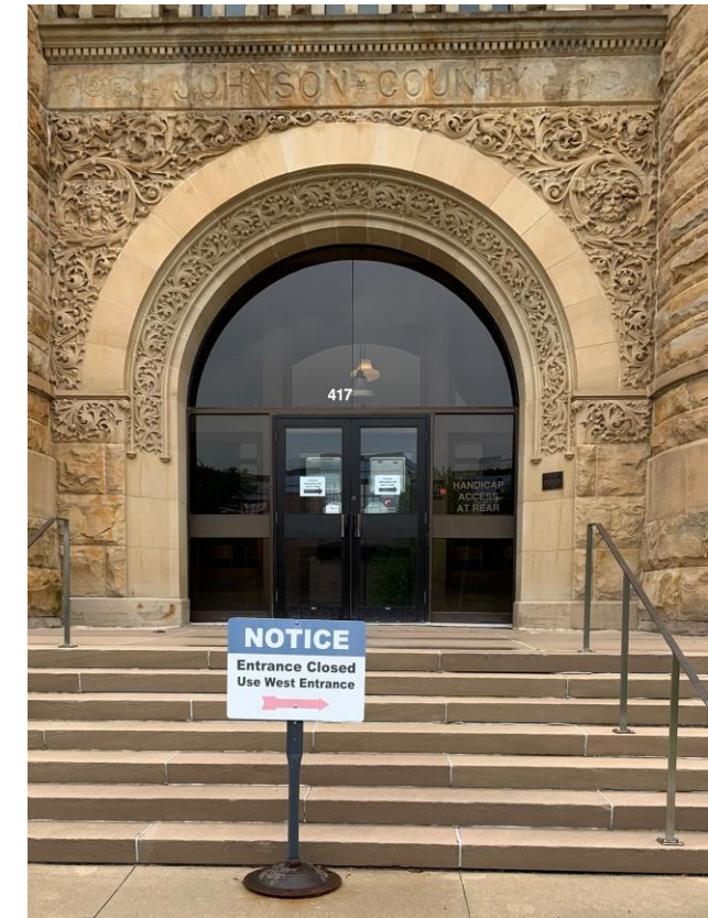
Pedestal sign at former east entry.
