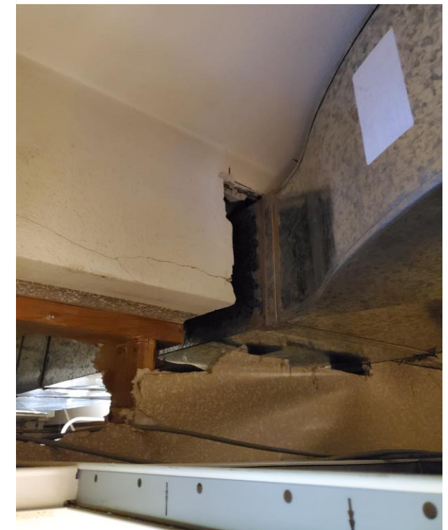
Duct penetration through wall above ceiling.
