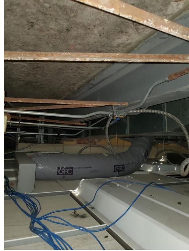
Ceiling plenum underneath second level.
