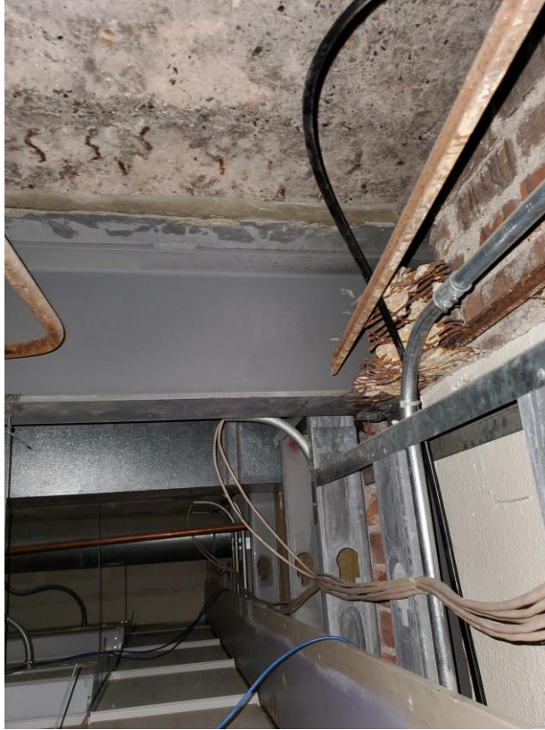
Framing and floor underneath second level.
