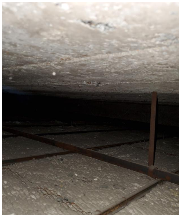
Ceiling plenum space and plaster ceiling.
