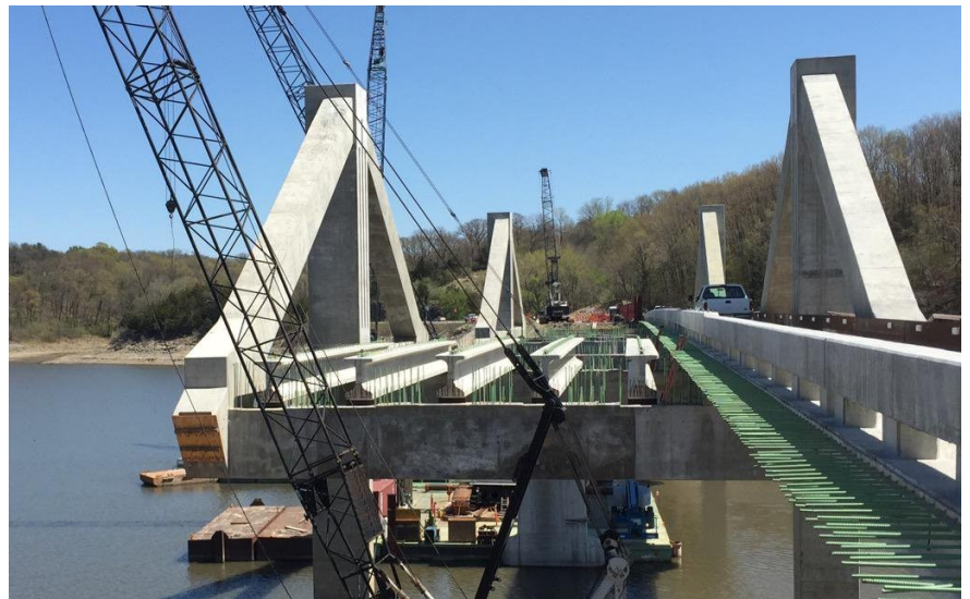
Mehaffey Bridge construction
